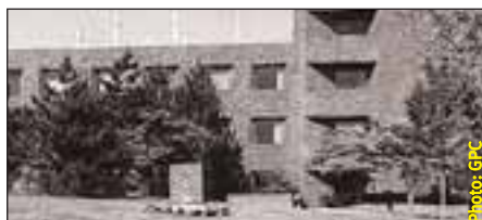
Locked up soon: GPC facility in Waltham, Massachusetts.
